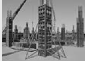
Column formwork
