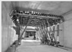
Tunnel formwork
