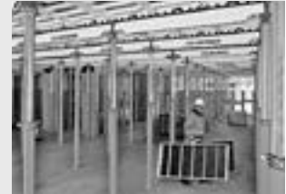
Slab formwork
