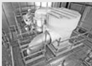
Working scaffolds industry
