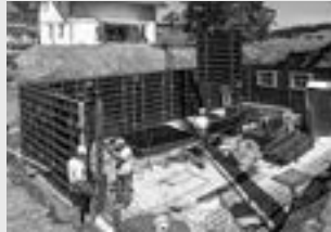
Wall formwork
