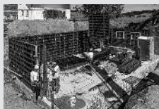
Wall Formwork
