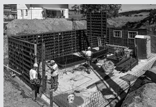
Wall Formwork
