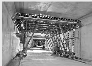
tunnel formwork
