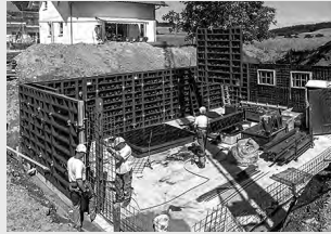
wall formwork
