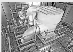
working scaffolds industry
