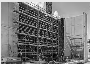
working scaffolds construction
