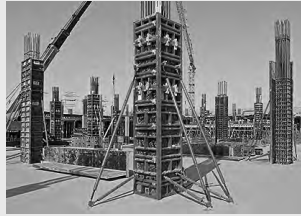
column formwork
