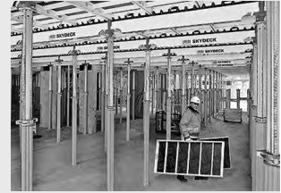
slab formwork
