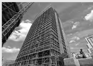
working scaffolds facade
