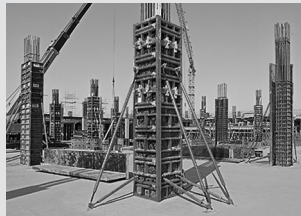
Column formwork
