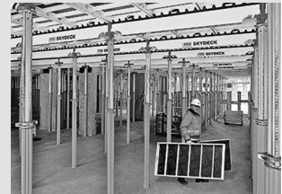
Slab formwork
