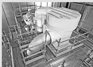
Working scaffolds industry
